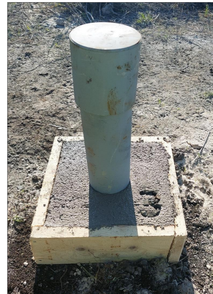
Figure 5 Lockable steel cover at borehole BH-3
