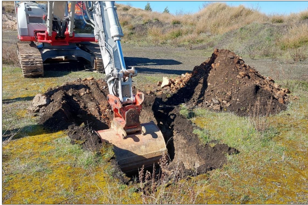
Figure 3 Excavation of trial pit TP-5
