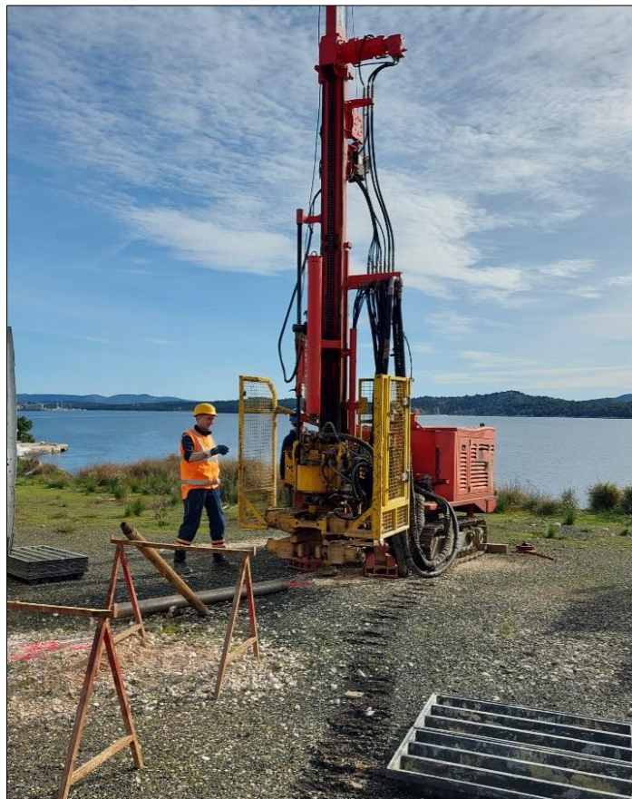
Figure 4 Drilling at borehole BH-4
